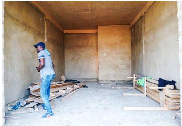
Enyinnda Shop interior – Plastered
