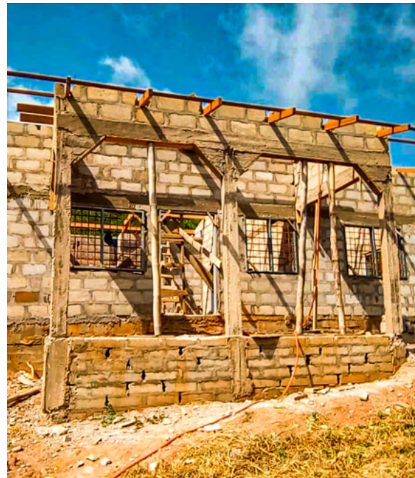
Work in Progress – Front Elevation
